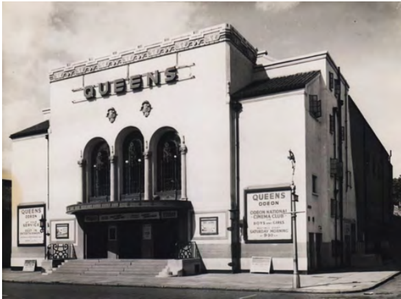
Exterior of the Queens (courtesy of 'Cinema Theatre Association Archive')
